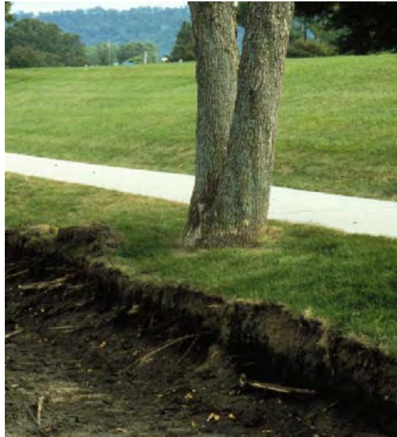
Figure 6. Severing roots decreases support and increases the chance of failure or death of the tree.
