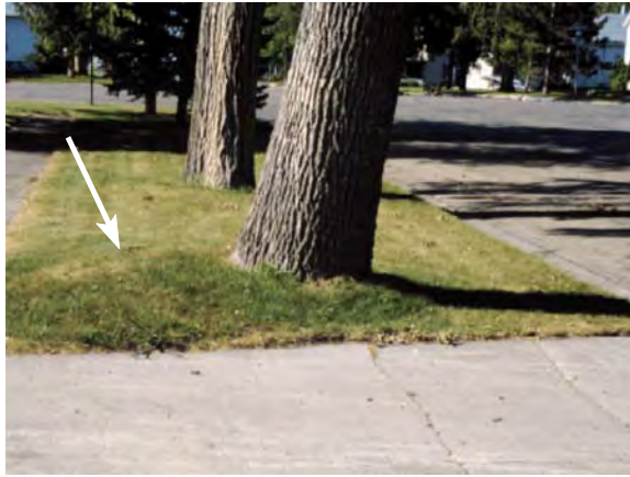
Figure 7. The mound (arrow) at the base of this tree indicates that the tree has recently begun to lean, and may soon fail.
