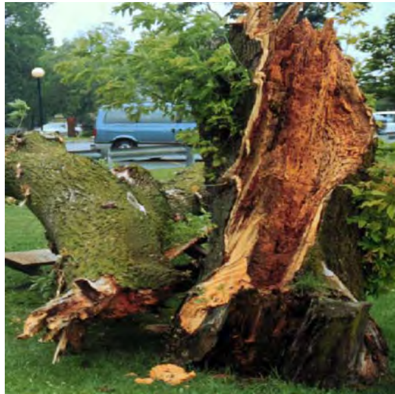
Figure 4. This seriously decayed tree should have been evaluated and removed before it failed.
